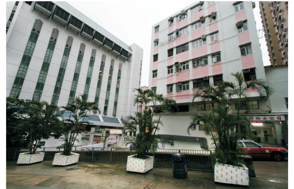
GIC7 Shek Tong Tsui Municipal Services Building
